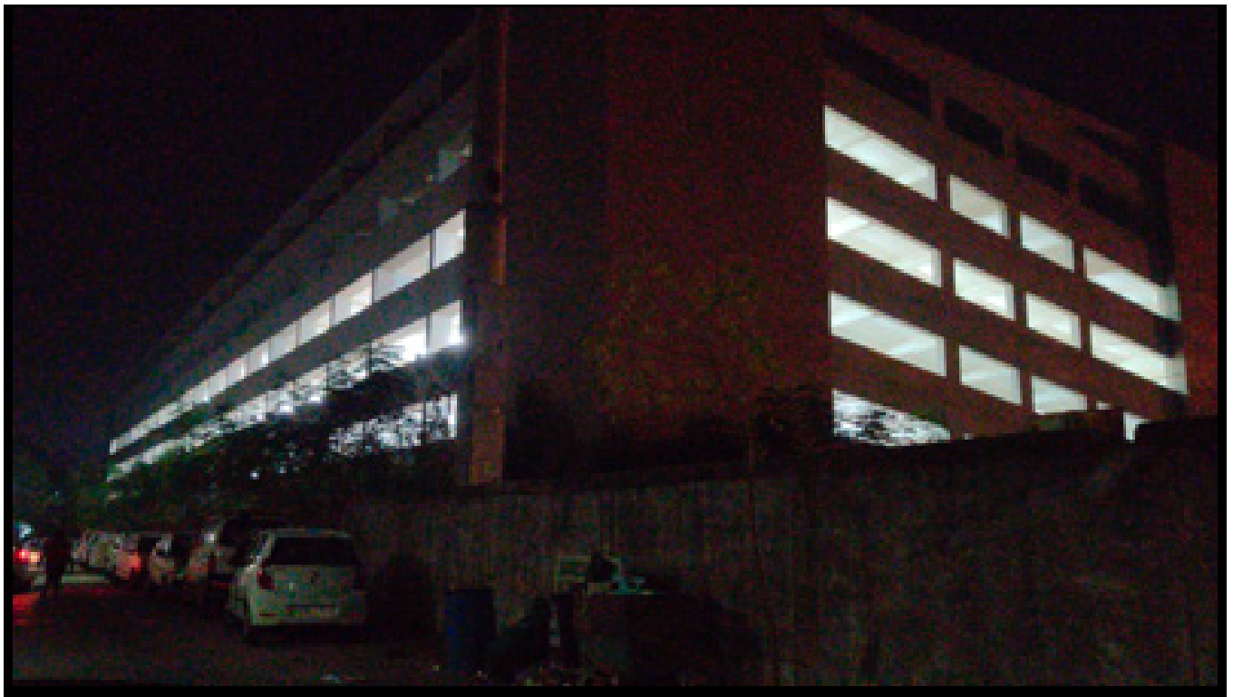
Figure 19: Parking lot in Surat converted in to COVID-19 care facility
